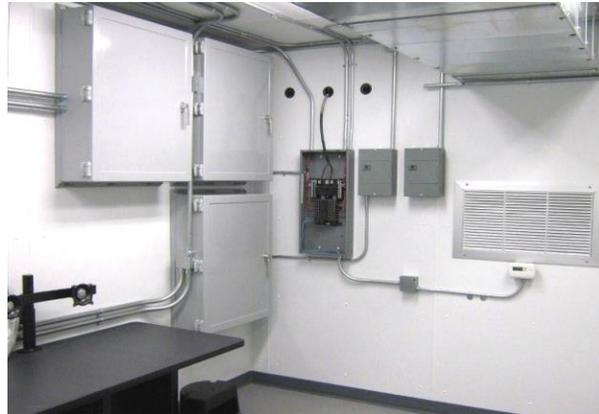
*Figure 2. Blast-resistant modules with ballistic up-armor are used to secure the SCADA nodes at each power plant from the harsh environment and terrorist attacks.*
